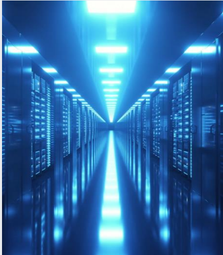
WIRELESS DATA CENTER
